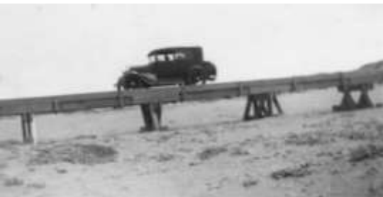
Left: The same car as seen above, driving over a trestle that enabled cars to cross the sand dunes.
