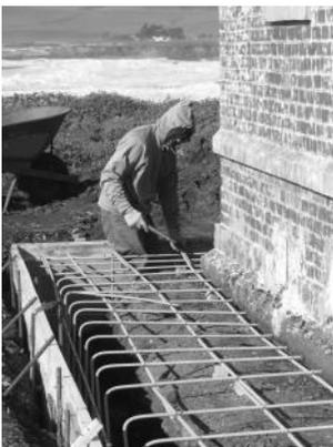
Above: Dan Murphy, working on rebar in the perimeter curbing.
