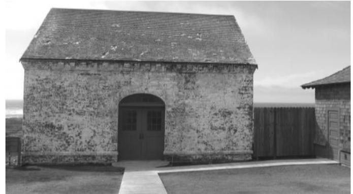
Above: Completed sidewalk replicates the original concrete walkway constructed in 1909 to connect the fog signal building and blacksmith shop.
