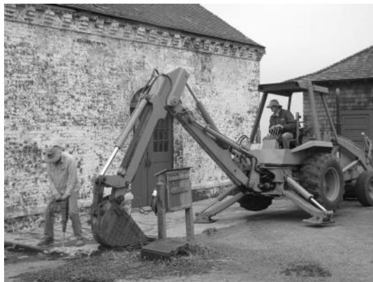
Above: The concrete apron in front of the fog signal building was removed. David Cooper is using the jack hammer, Dan Murphy is operating the backhoe.
