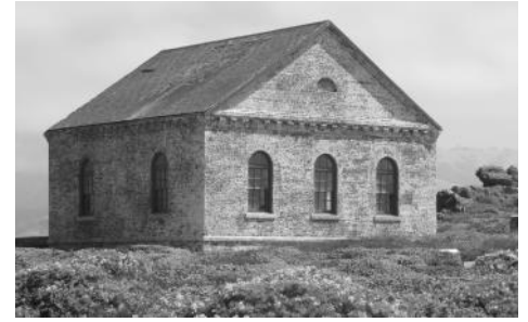
Fog signal building restoration in progress 2010-2014, partially complete.
